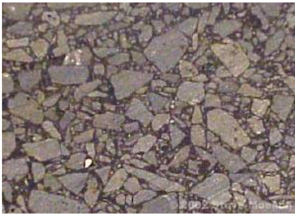
Typical Stone Matrix Asphalt surface.
