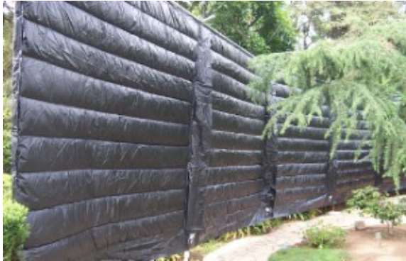
Acoustical Blanket used along Highway in California
