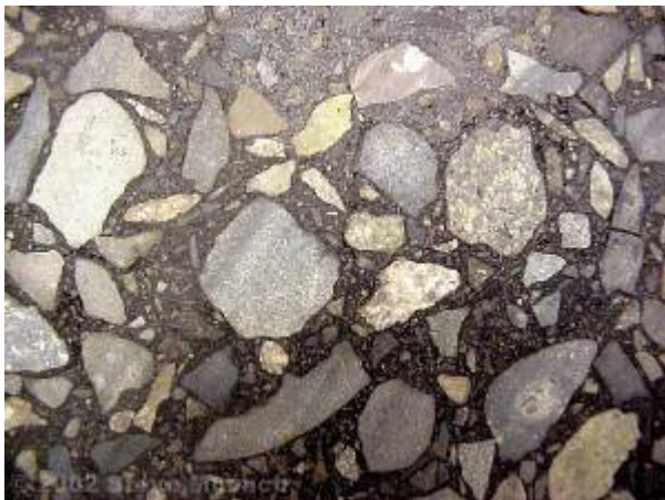
Typical DGA surface
