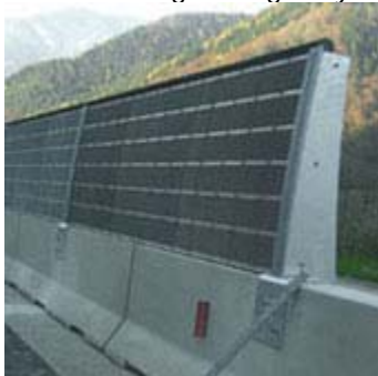
Calm Tracks mounted on Jersey Barrier
