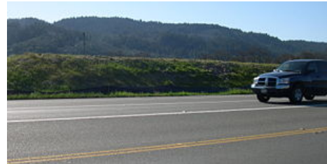
Low Roadside Soil Berm
