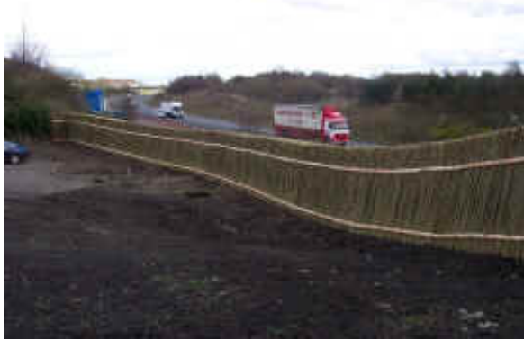
Green Barrier Under Construction
