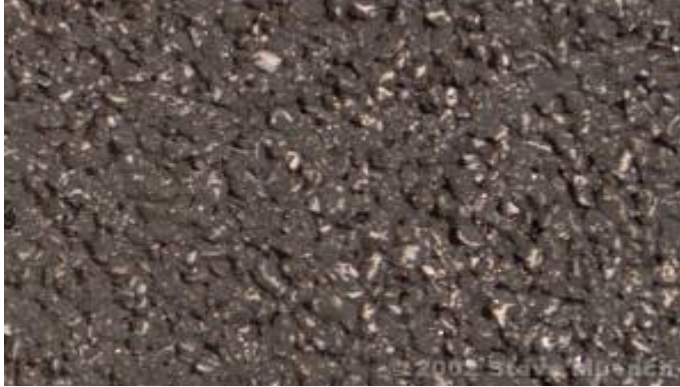
Typical Open Graded Asphalt Friction Course Surface
